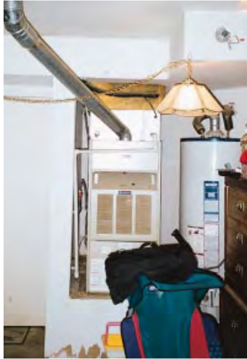
Figure 21. As a matter of life safety, combustion appliance vent pipes must have proper clearance to combustibles. The guidelines are usually stamped right on the appliance itself.
