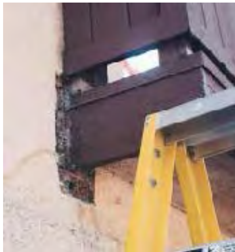
Figure 12. Framing protrusions, such as handrails (left) and cantilevered joists (right), are difficult to flash properly, inevitably leading to moisture intrusion, cracked stucco, and decay in the structure below.
