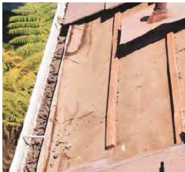
Figure 8. A raised fascia board (illustration) requires a heavy metal flashing or cant strip to ensure that runoff passes over the edge. Otherwise, water will pond, as in the photo, resulting in leaks and rot in the eaves.
